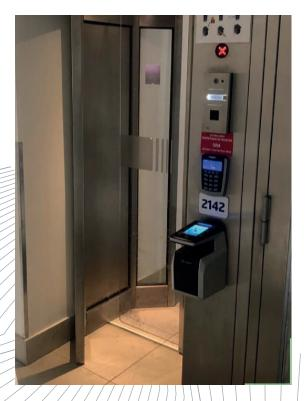
In order to avoid any physical contact with the devices, for user convenience as well as for hygienic considerations, it was decided to deploy a contactless biometric technology.
